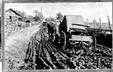
Typical Spring condition of soft-surfaced roads
